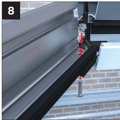
8 Using nuts and bolts (SHBC001S - found in BURBOX), locate each hip bar and secure to radius end by hand tightening nuts.
