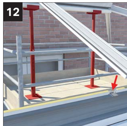
12 Depending upon the lantern size and options requested, fit hub end transom bar and / or side transom bars. If specified on the job, remove nuts from bolts in transom position and fit transom bar over bolts. Re fit nuts and hand tighten. Check that ridge is level and fully tighten nuts on all bars.
