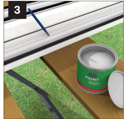
3 Finally, apply an air drying top coat with a fine brush.
